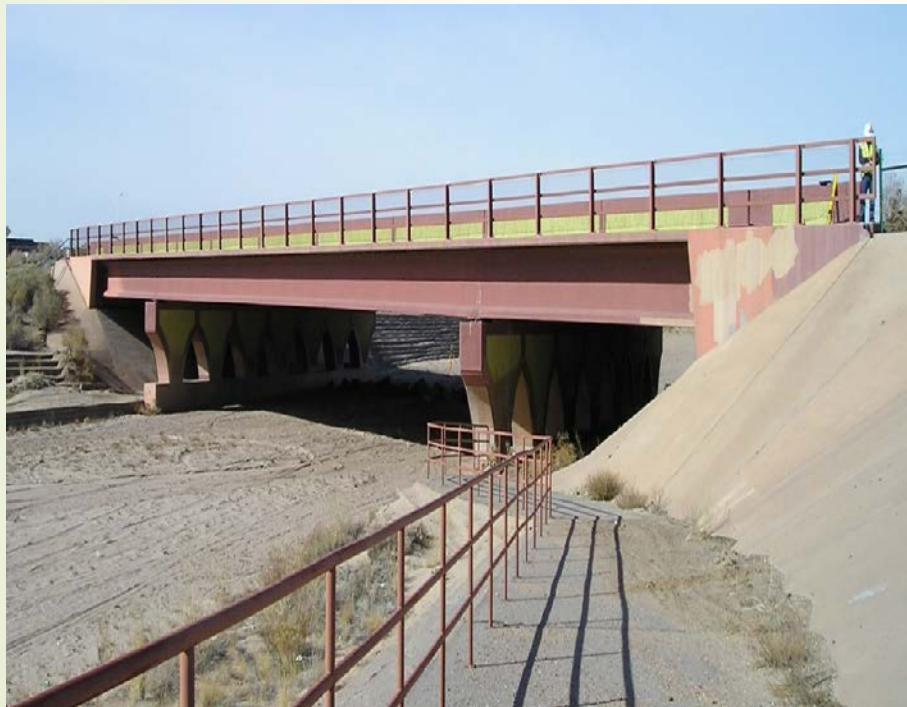
Bridge over the Calabacillas Arroyo
