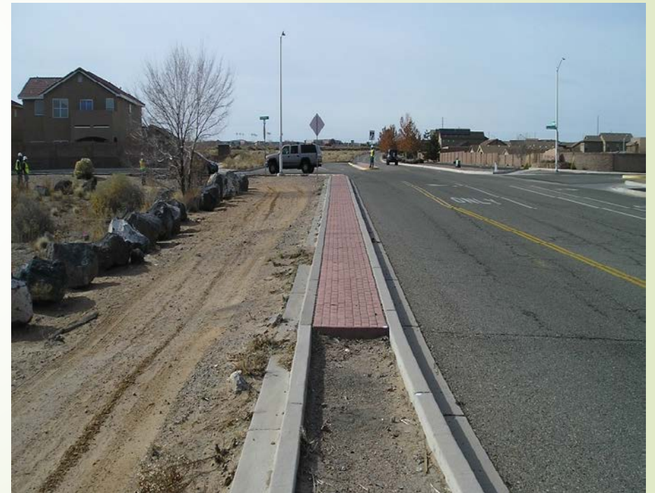
Median at Kayenta St. Facing East
