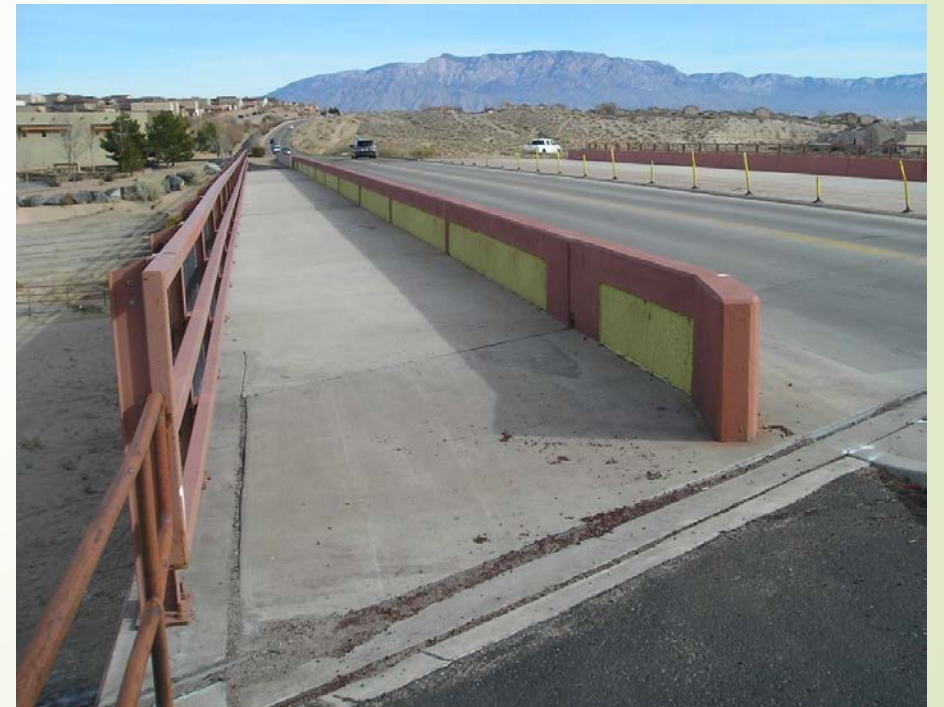
Pedestrian Access on North Side of Bridge
